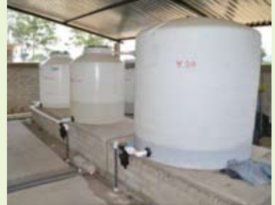
Fertilizers tank center at the Head control
