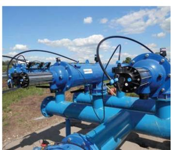
The control valves enable automatic operation of the irrigation system, as well as regulation of pressures according to the hydraulic design.
