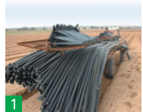
Laying out an Amirit system
